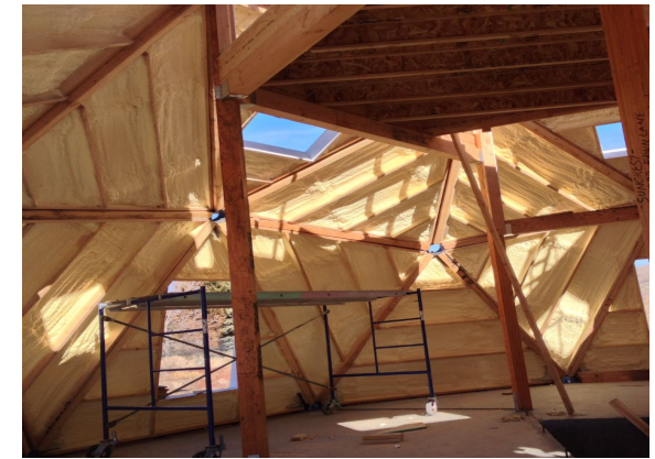
Second row of panels connect to the central core, which locks it all together.
