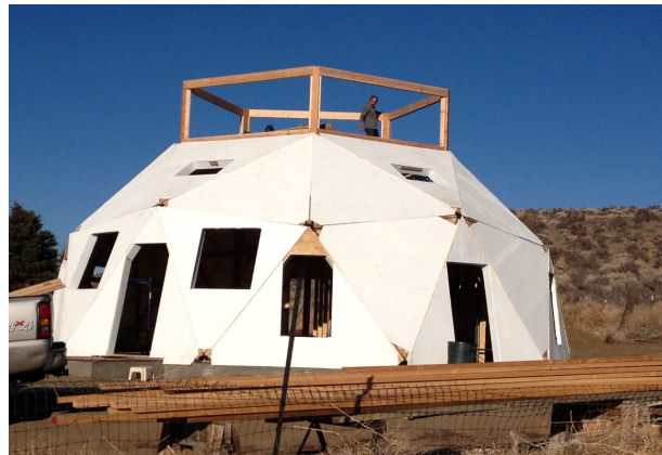
Symmetrical shape creates even load paths, resulting in extra structural stability
