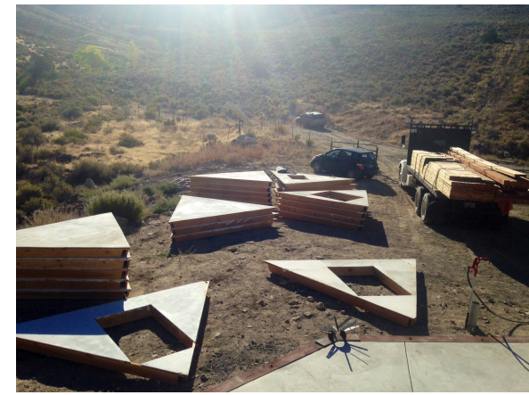
Triangular panels used for the exterior can be fabricated off site.
